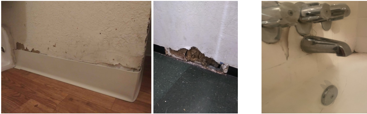
Figure 8: (Left to right) Dilapidation of internal and external baseboards; bathtub fixtures
