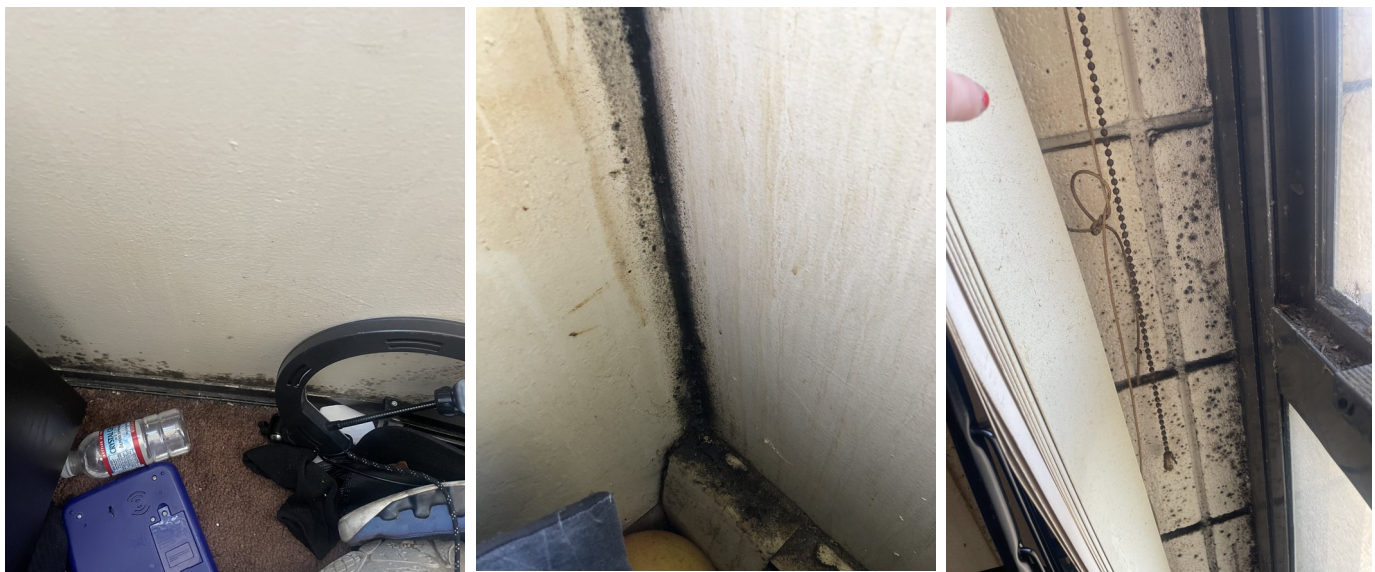
Figure 7: Mold on walls of a unit in building A
