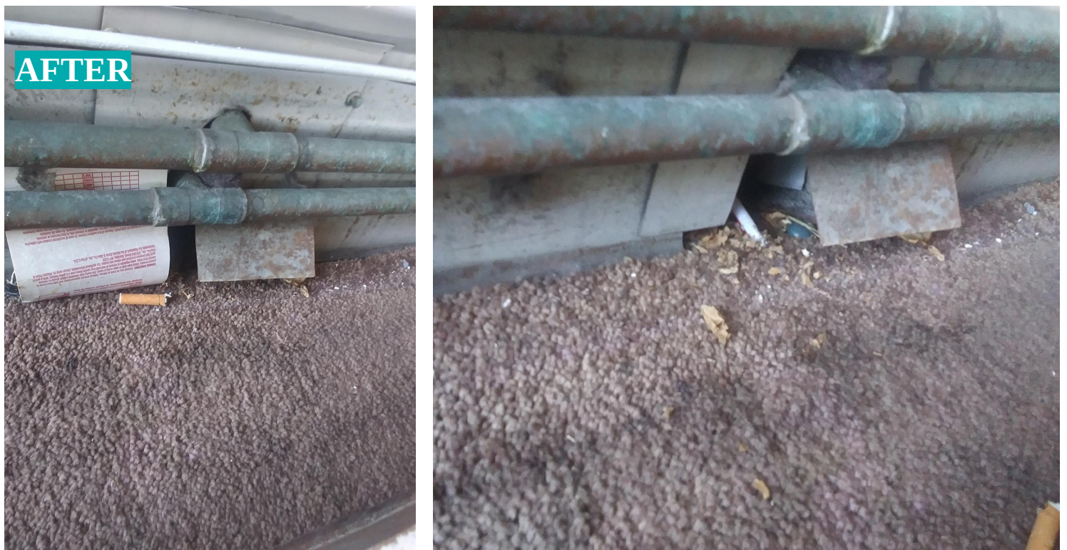
Figure 30: Mouse debris still present behind heating unit that was repainted without disassembly
