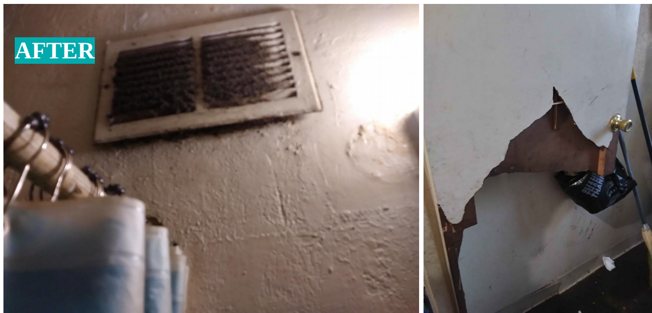
Figure 27: (Left to right) Bathroom vent in DL's unit left inoperable and covered in dust and grime during repair campaign; bedroom door still half broken off and not replaced by repair workers
