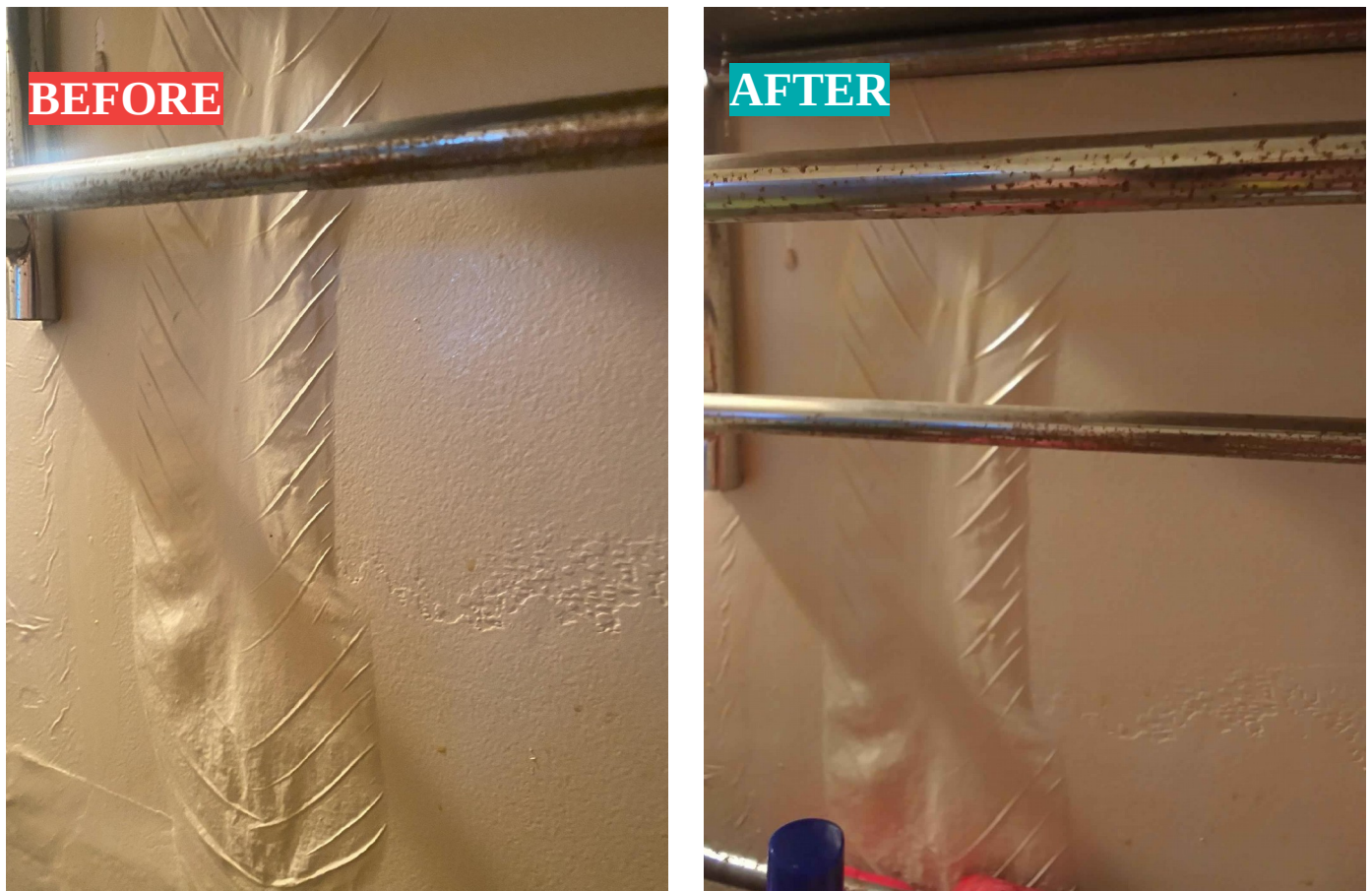
Figure 28: Bulge in bathroom wall before (left) and after (right) repairs at LJ's unit
