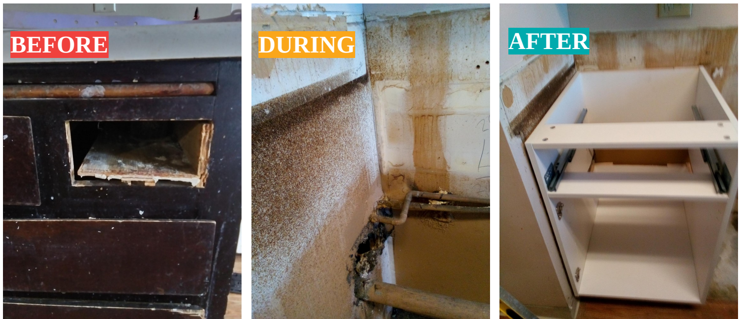
Figure 29: Kitchen cabinets before (left), during (middle) and after (right) repairs of kitchen cabinetry at EJ's unit. Note dirt, grime, and corrosion left on wall beneath the replacement unit.
